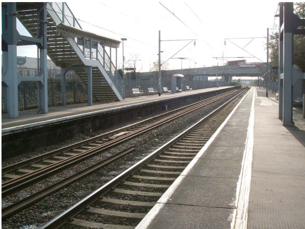
Figure 5.5 Angel Road Station
