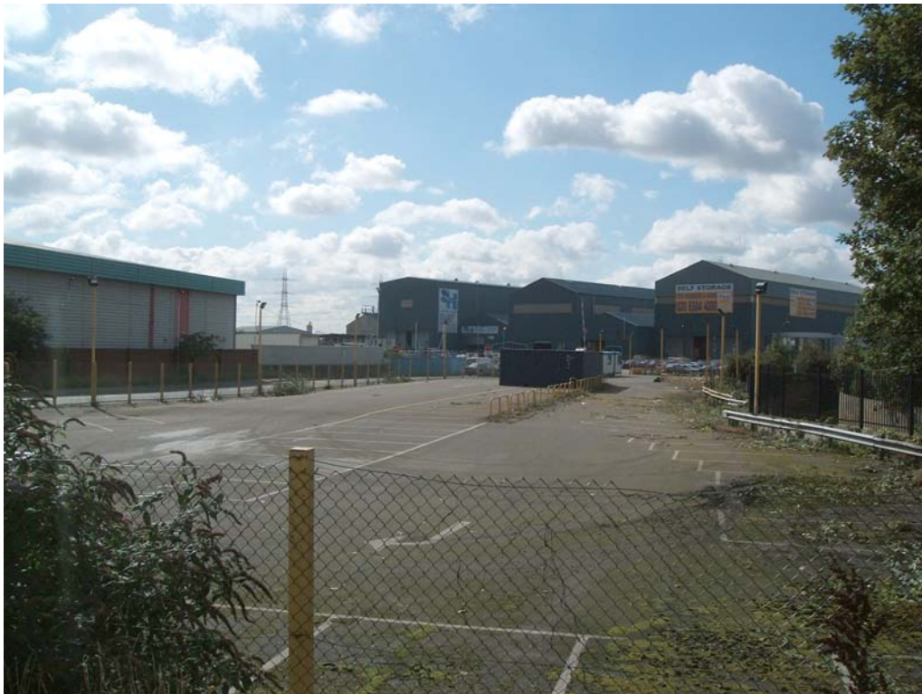
Figure 7.6 Former BOC premises
